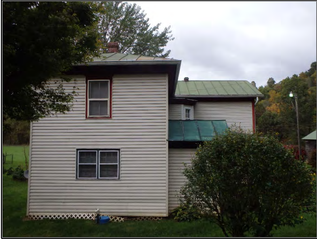
Figure 14. Rear elevation of the rear ell, facing northeast.
