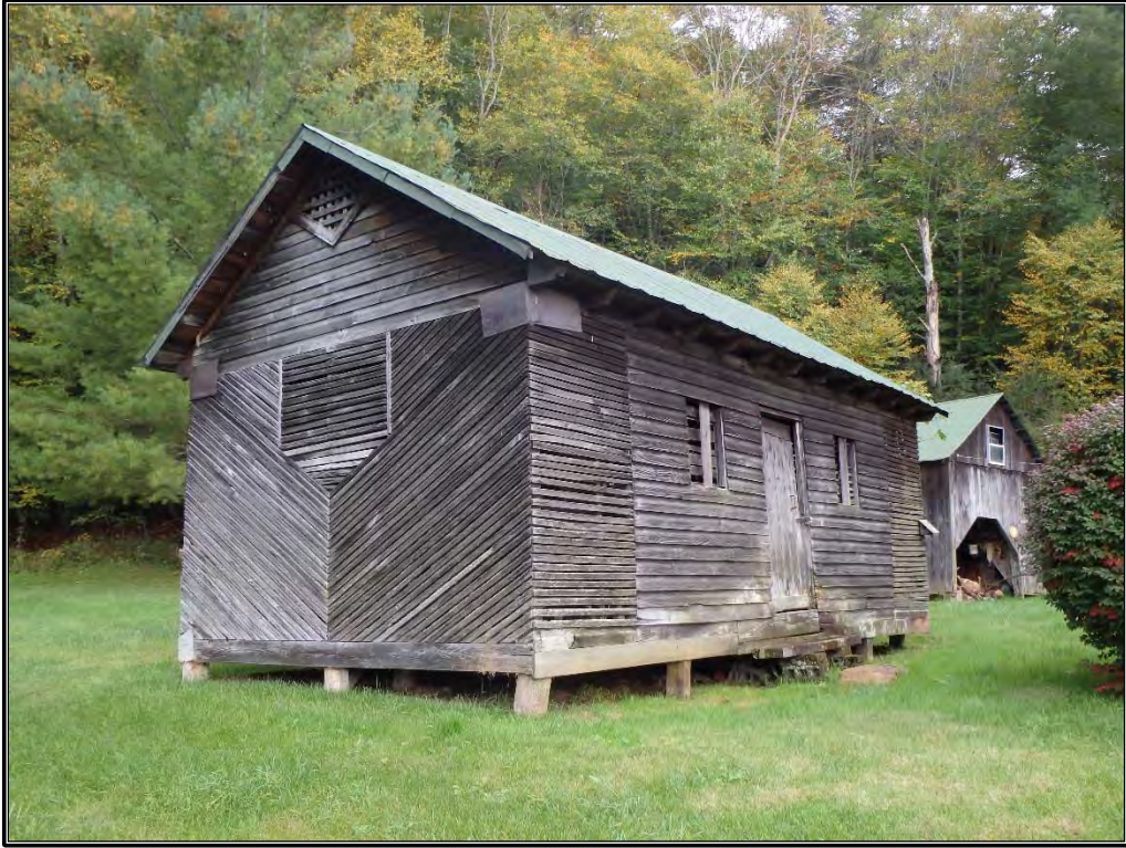
Figure 18. Granary, facing south.
