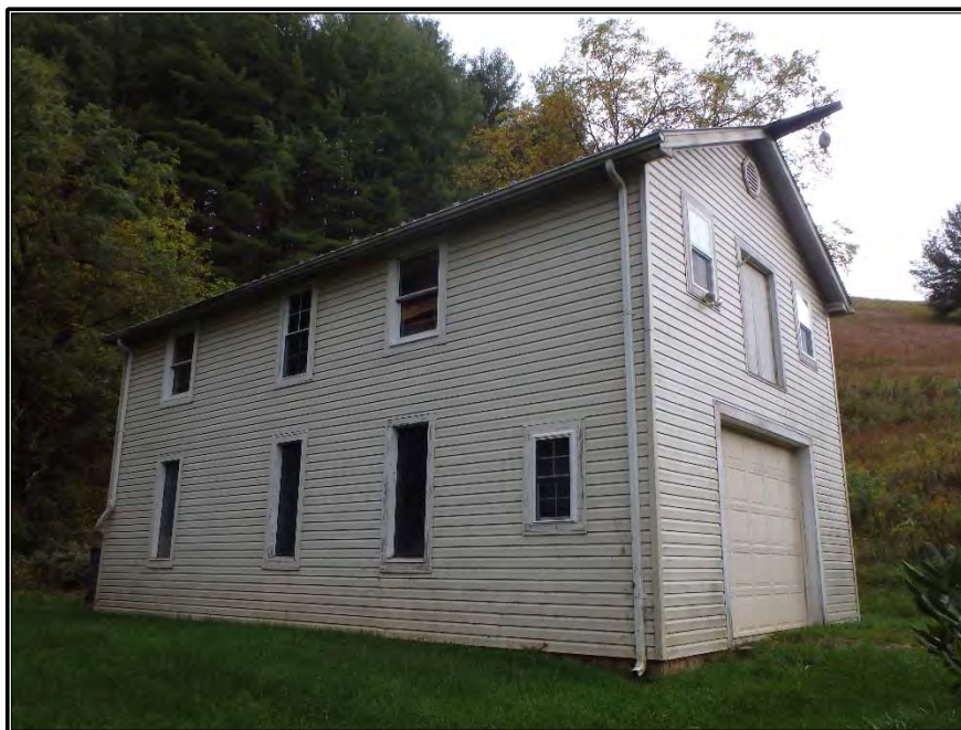
Figure 21. Modern Garage, facing west.
