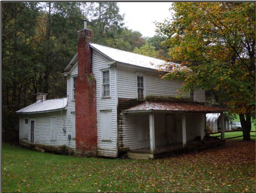
Figure 25. Comparative example, the Frank Seagraves House (AH 191), located at 1538 Little Helton Road, facing south.
