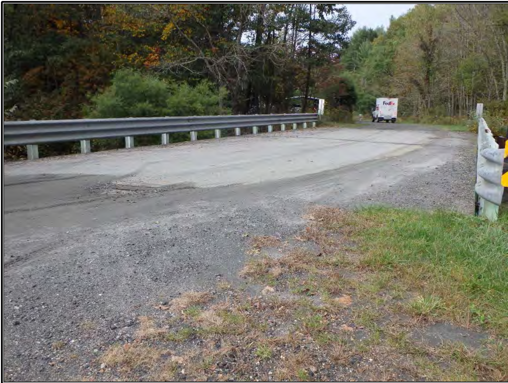
Figure 8. Overview of Bridge No. 288 over Helton Creek, facing west-northwest.
