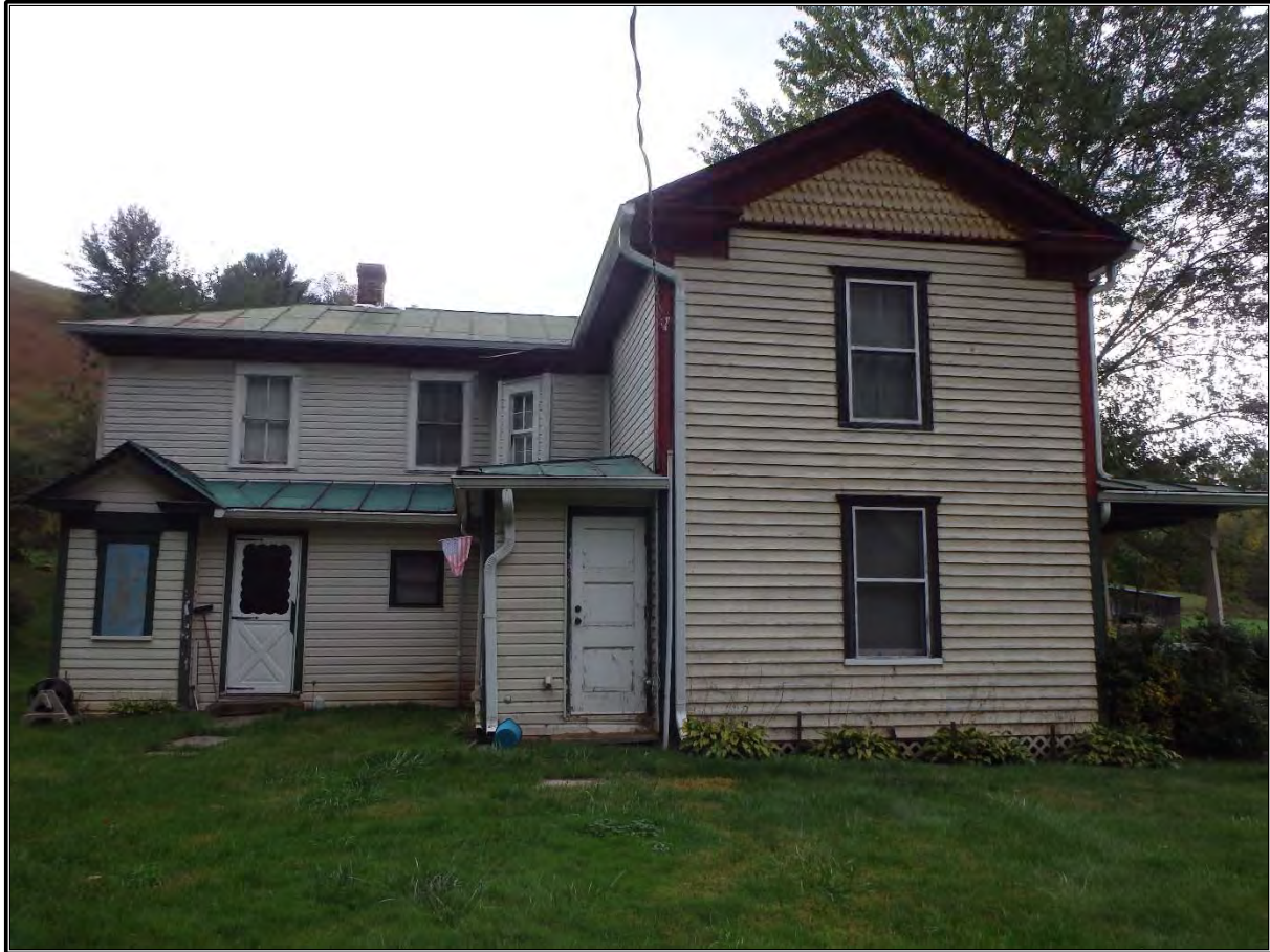
Figure 13. Southeast (side) elevation, facing northwest.
